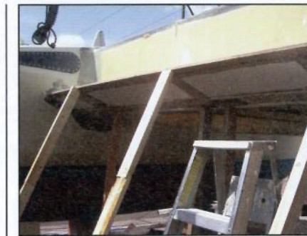
Installing new panels with 2x4 props holding them in position.
