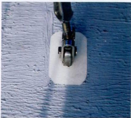
Chainplates that pass through the deck are a common source of leaks.
