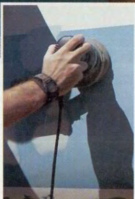
Photos 2–3: Spread the filler evenly over voids and overfill so the dry surface can be sanded smooth
